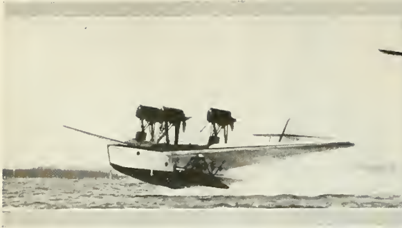
Rohrbach Romar with three B.M.W. water-cooled engines
